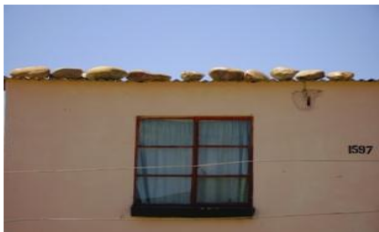
Figure 3: Unsecured Roofing. Hankey, Eastern Cape. Source: Khanya-aicdd, 2008: 10.
