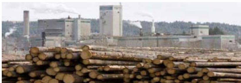
Figure 48 West Fraser Timber, Quesnel, B.C. Credit- www.cbc.ca
