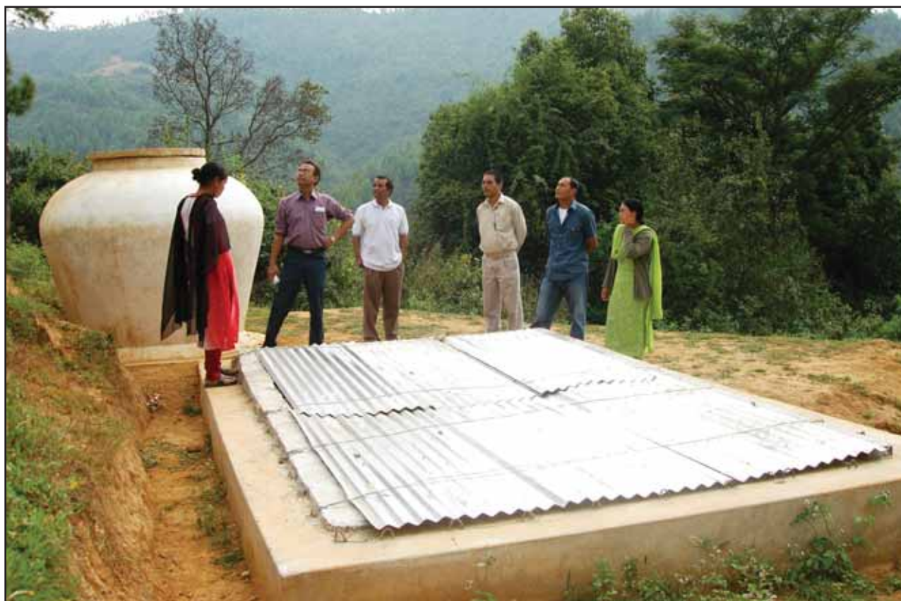
Figure 8: Modified Thai Jars and Ferrocement lined tanks for water storage under the MUS projects.
