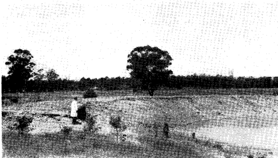
Fig. X showing portion of a farm dam constructed for the purpose of storing run off during periods of heavy rainfall. Dams such as these can be developed on many coastal farms to serve irrigation plants when other sources of fresh water are not available.
