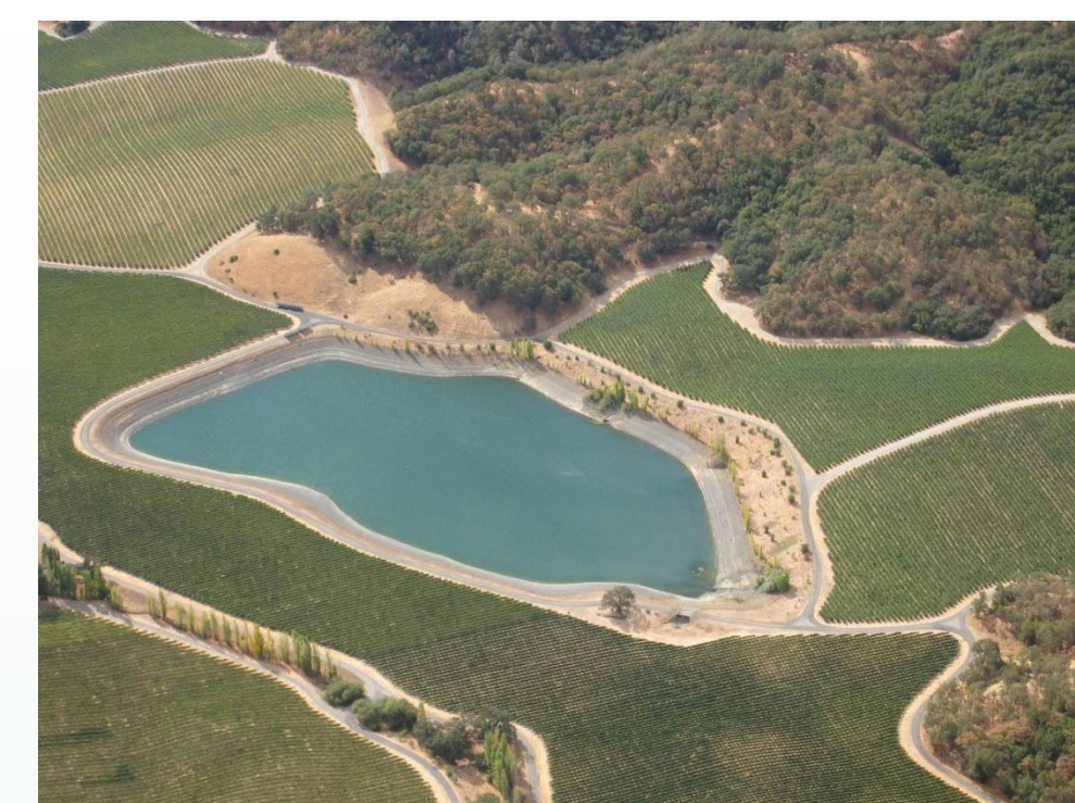
Figure 2: An onsite reservoir located next to vineyards
