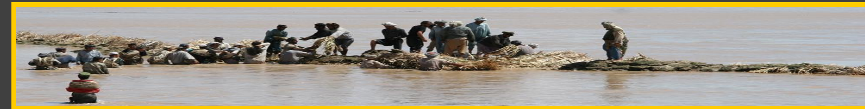
Afghan villagers construct a sod diversion dam (above). These dams are washed out several times a year, especially during the periods of high flows (see hydrographs, top). The goal of this project is to determine the most economically-optimal method of managing these flows. (Fipps, 2009)
