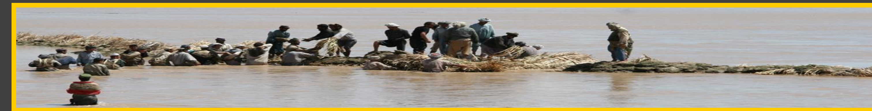
Afghan villagers construct a sod diversion dam (above). These dams are washed out several times a year, especially during the periods of high flows (see hydrographs, top). The goal of this project is to determine the most economically-optimal method of managing these flows. (Fipps, 2009)
