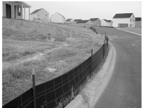
Figure 1. Use of a Silt Fence on a Residential Lot Under Construction in Study Area
