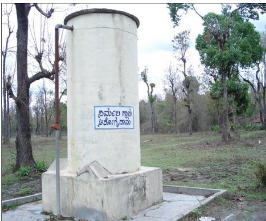
Drinking water facility in tribal village
