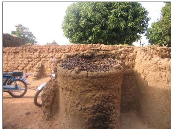
Figure 4: Shea Drying Oven, Cercle de Dioila, Mali (Perakis, Fieldwork, 2007)
