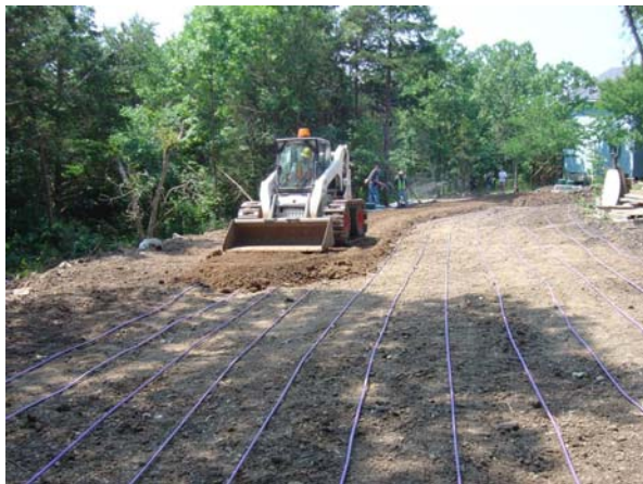
Figure 45. Drip Irrigation Installation
