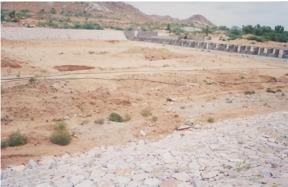
Check dam at Chigatagere separating the non-sand mining villages on left side from sand mining villages on right side, Gaurubidanur taluk, 2003
