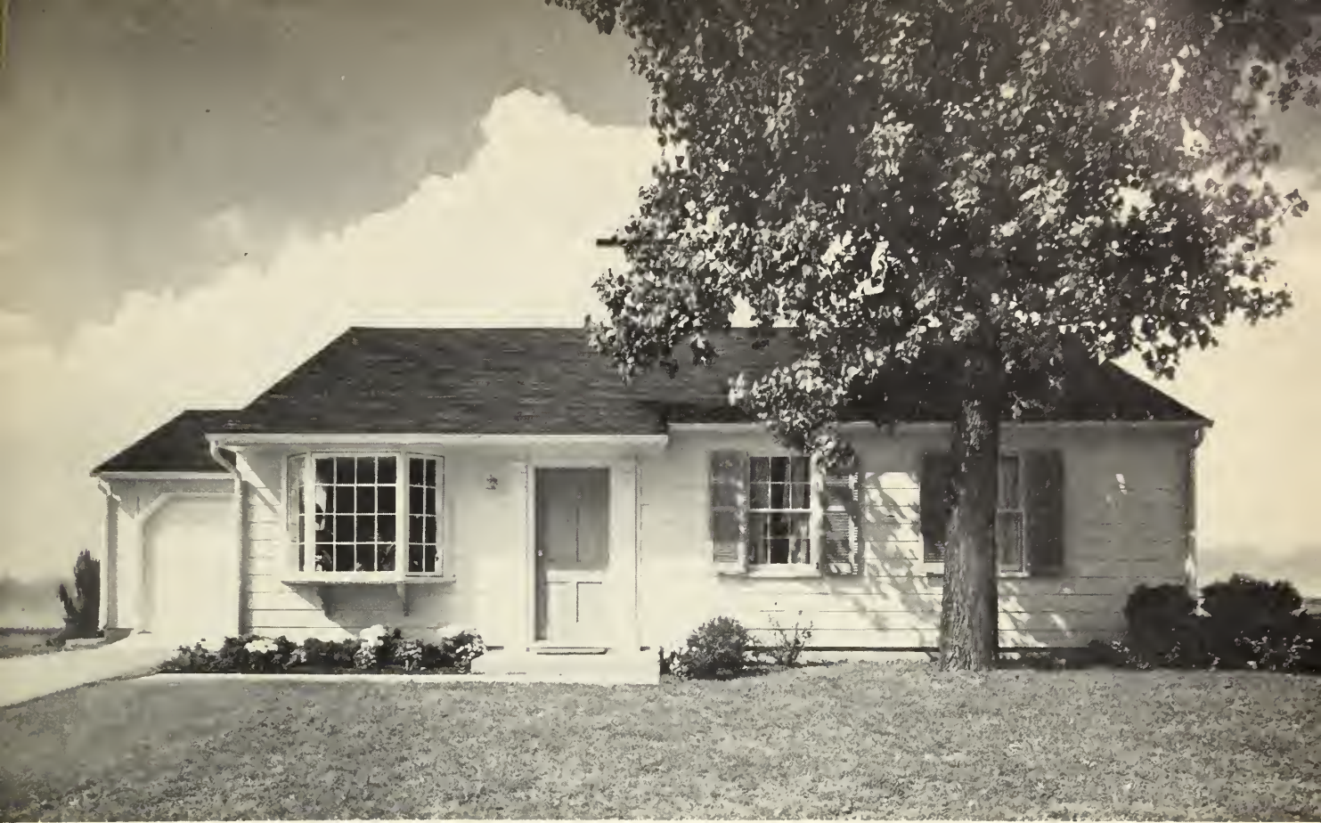
The factory house today cannot be distinguished from its custom-built counterpart.
