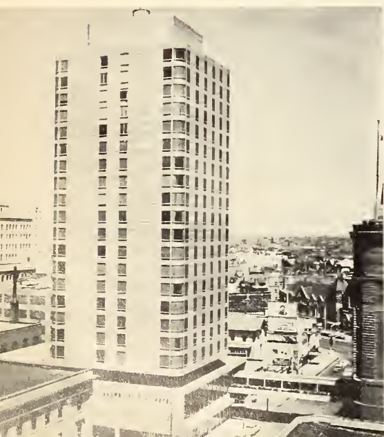
Left: This hotel in Denver has honeycomb-core wall panels faced with steel, and an outside ceramic coating. Right: The beauty and utility of good wood furniture is timeless.
