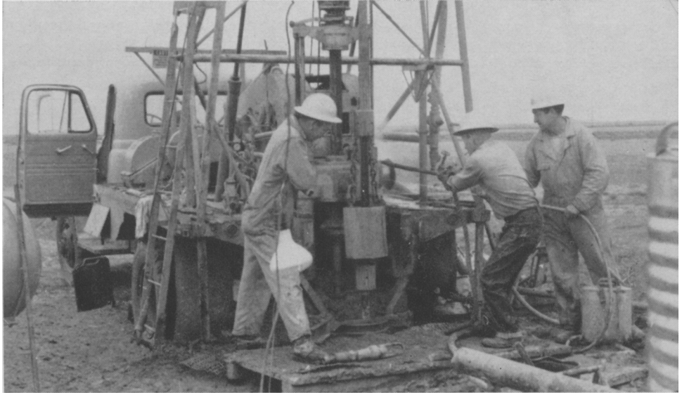
Fig. 3. Drilling for substrata core samples.
