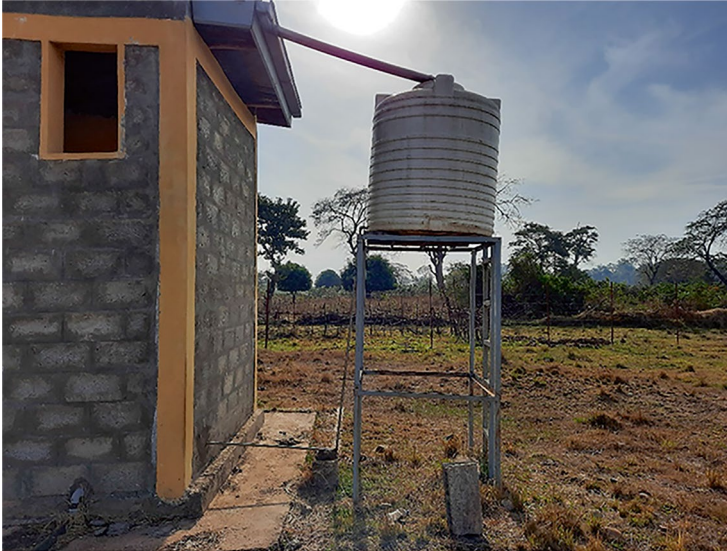
Fig. 15.3 Rooftop water harvesting using water tanks in Oromia region, Ethiopia. (Photo Credit: Desalegn Tegegne)
