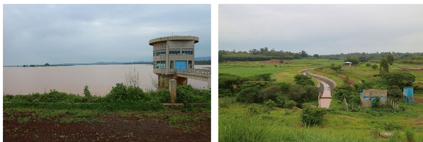
Fig. 15.2 Formal community irrigation scheme, Koga irrigation scheme, Ethiopia. (Photo credit: Desalegn Tegegne)
