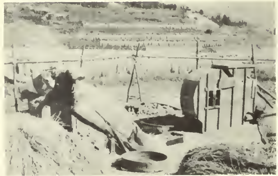
Figure 2.-- Manually operated threshing machine
