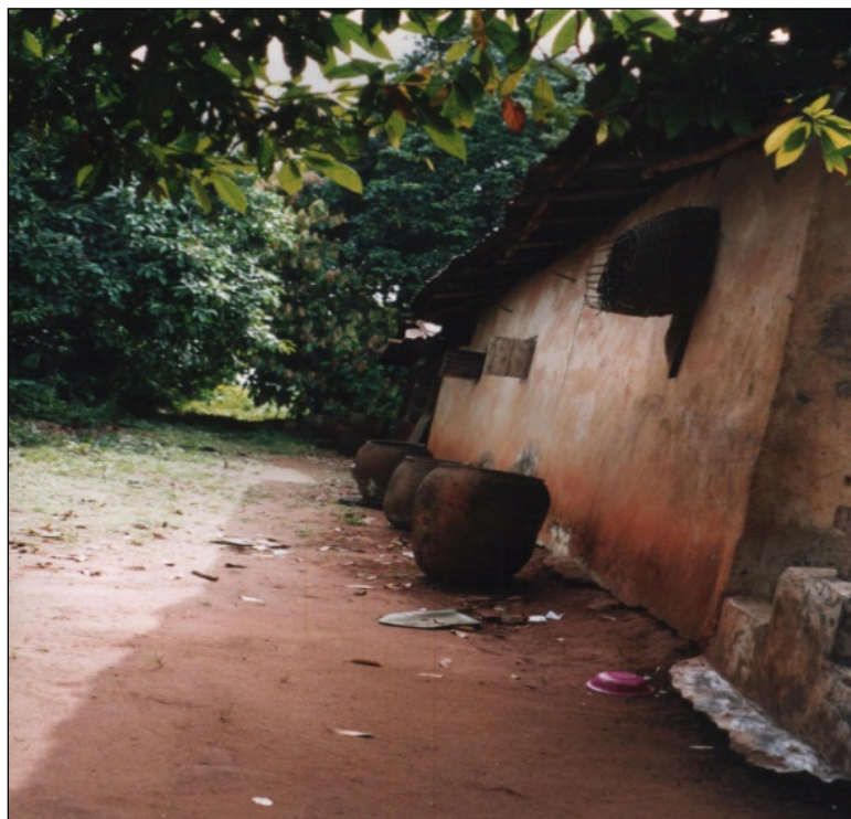
Photo 1. Rain Water Storage Facility in Uzanu
