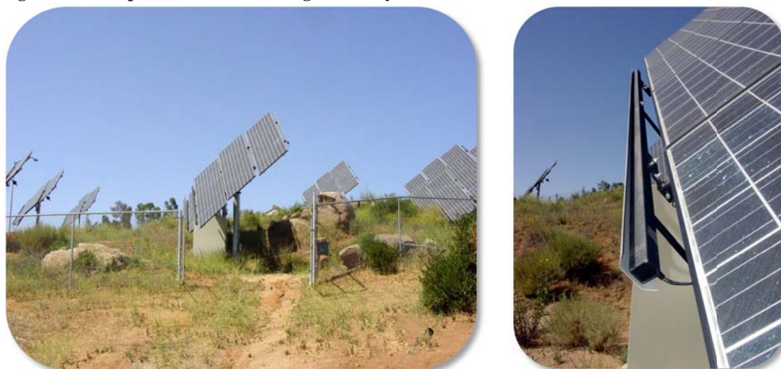
Figure 7. Example of Passive Tracking PV Array
