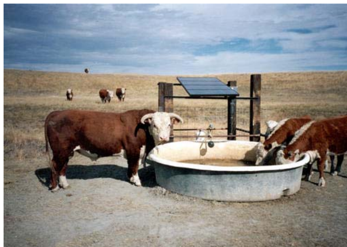
Figure 19. Solar-powered water pumping station. Source: NREL PIX.
