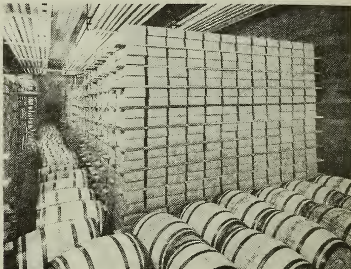
Figure 4. - Storage temperatures of approximately 0° F. are recommended. For certain products they should be even lower. Cartons must be stacked away from walls and ceilings and laid upon strips of wood so the air flow will not be impeded. For those not completely frozen, vertical spacing also is needed, as well as dunnage between every other layer. Barrels are laid down and rolled periodically to insure complete mixture of contents until frozen, after which they are stacked on end.
