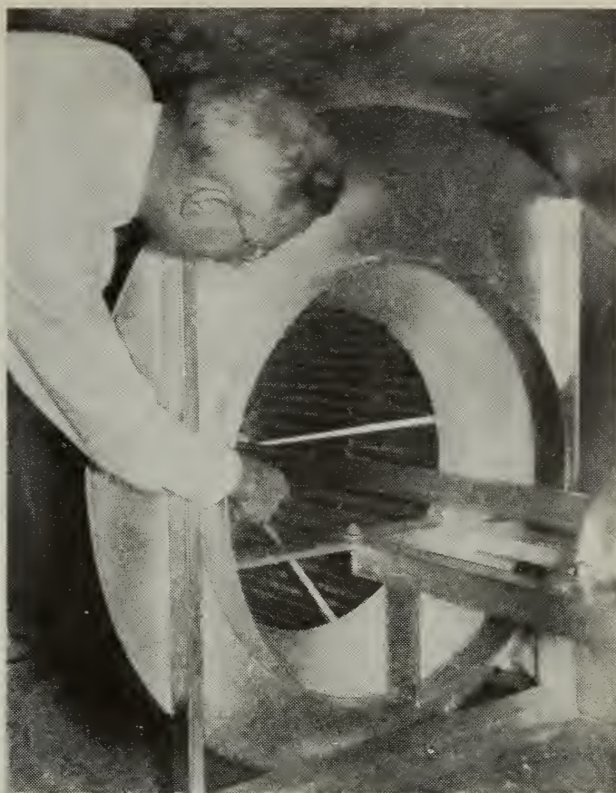
Figure 19. - One of four "squirrel cage" fans which supply 100,000 cubic feet of air per minute. The air circulates over the product to be frozen and then passes through a large coil in which is ammonia at 50^{\circ} F. below zero. The result is a temperature of 40^{\circ} F. below zero for freezing purposes.
