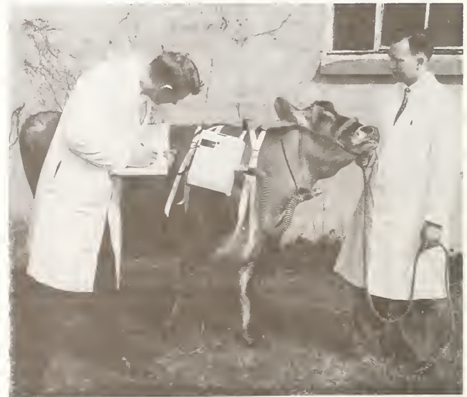
A portable respirator, developed in mid-1960's at BARC is tested by scientists D. R. Waldo and W. P. Flott. This apparatus was developed to determine the energy requirements of cows while on pasture.
