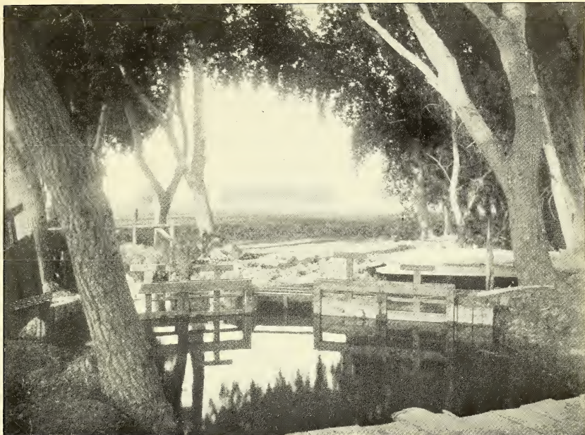
FIG. 1.—DIVISION GATE ON IRRIGATION LATERAL, NEAR ROSWELL, N. MEX.
