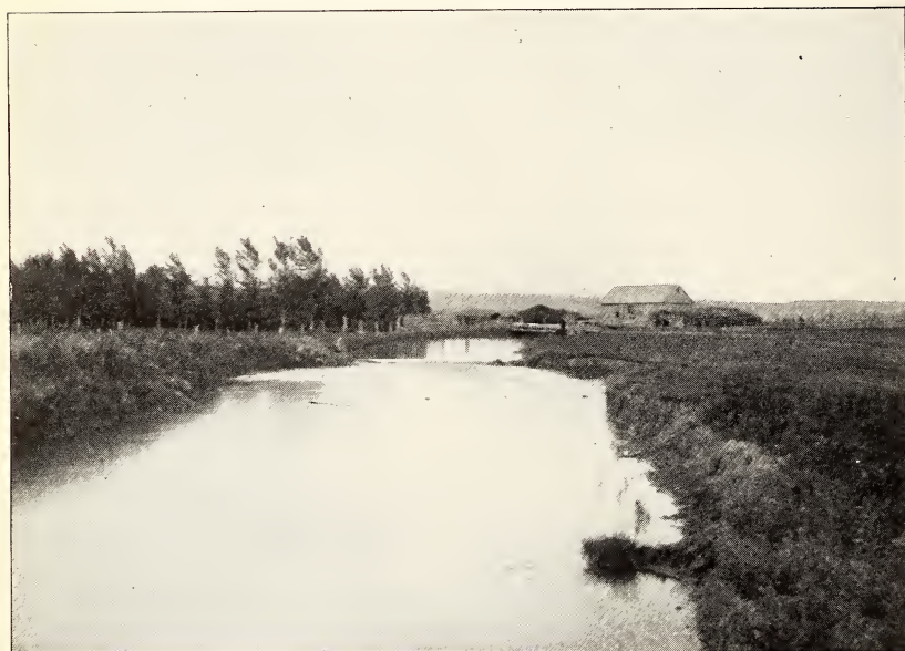
FIG. 2.—CANAL NEAR BILLINGS, MONT.
