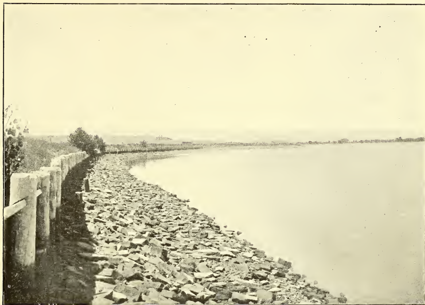
FIG. 1.—PILING AND RIPRAPPING ON EMBANKMENT OF CACHE LA POUDE.
