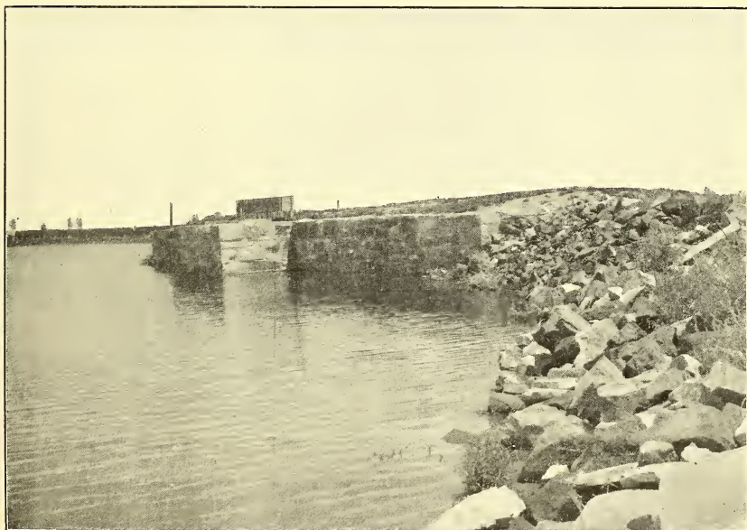
FIG. 2.—MASONRY GATE WELL, LARIMER AND WELD RESERVOIR.
