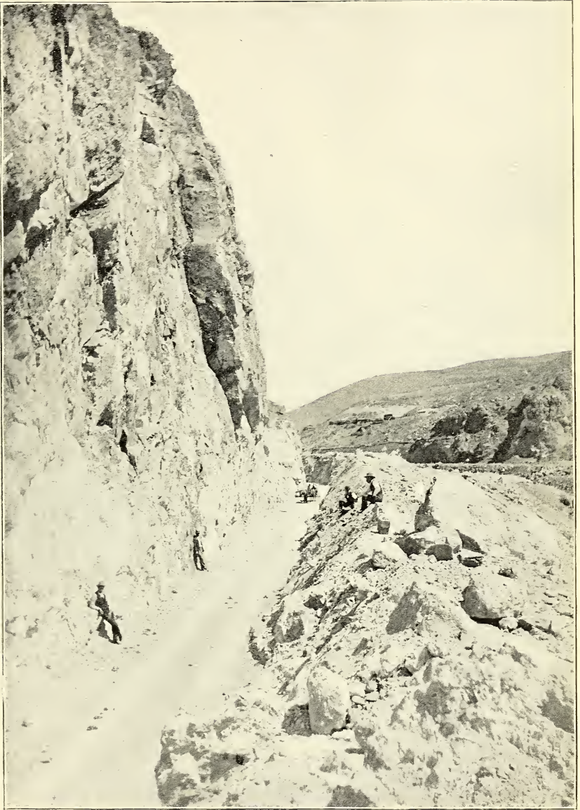
ROCK CUT 97 FEET DEEP, BEAR RIVER CANAL.
