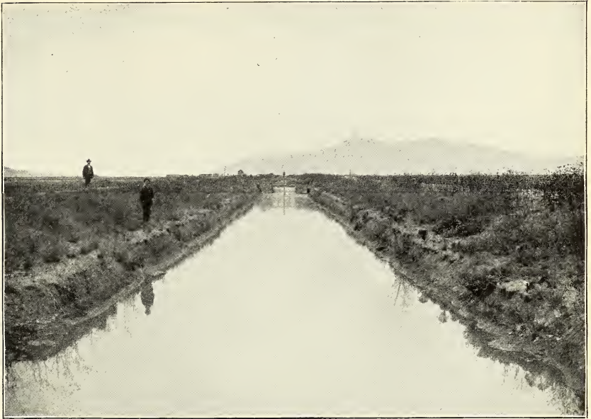
FIG 1.—BEAR RIVER CANAL, LOOKING NORTH SHOWING DROP.
