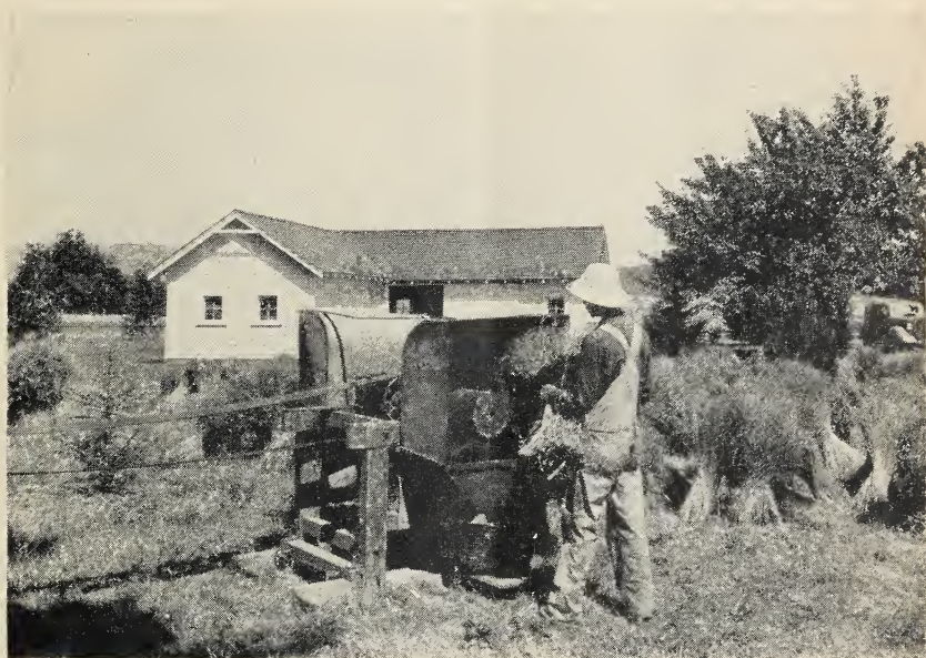
FIGURE 13.—Deseeding flax straw from experimental plots with a "whipper."
