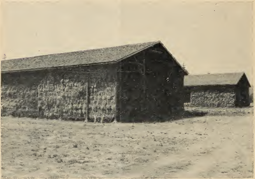
FIGURE 3.—Typical flax-straw storage sheds with north end and east side open; the prevailing wind during the rainy season is from the southwest. Such sheds are usually 56 feet wide, 240 feet long, and 18 to 20 feet high to the eaves.
