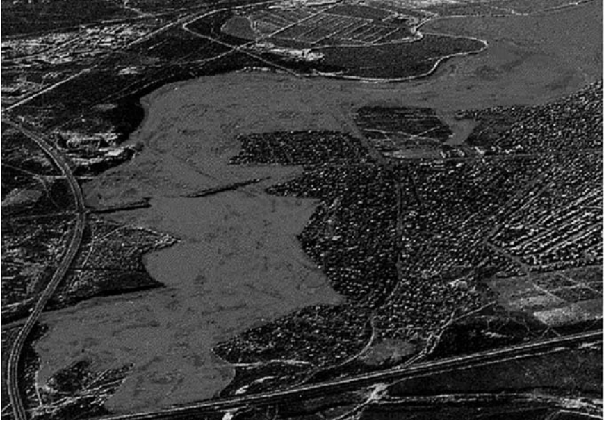
Figure 1: Aerial view of Soweto-on-Sea relative to the Chatty River, some tarrred roads and the 1:50 year floodline
