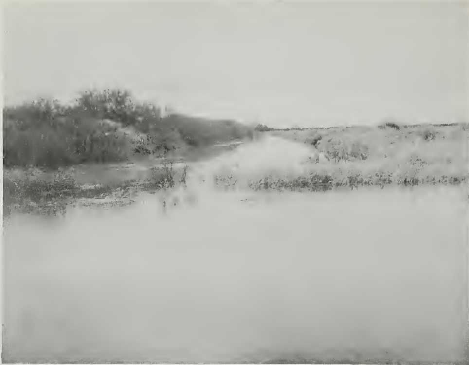
Existing drainage ditches lack depth and capacity to meet present requirements (top) and are in need of maintenance (bottom).
