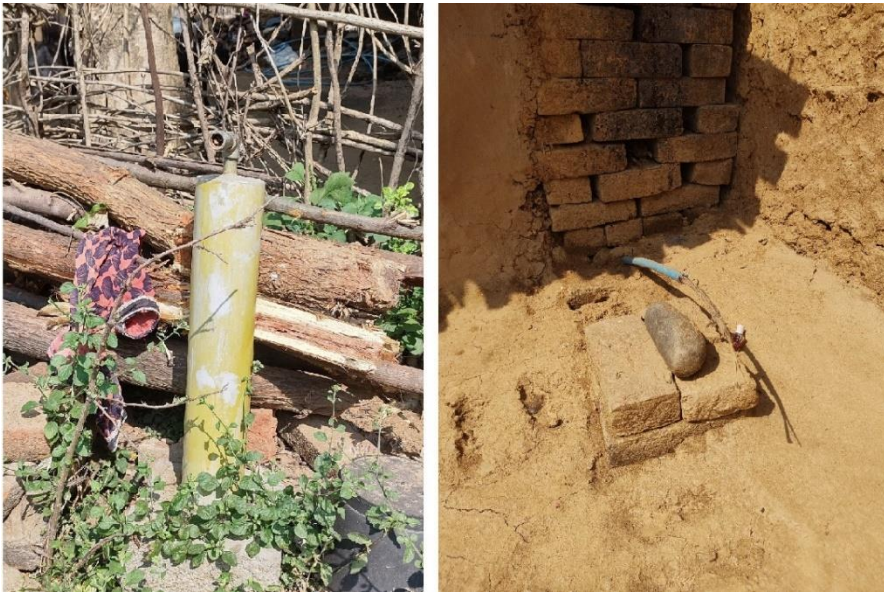
Figure 6: Abandoned Tap Connection in Ward 3, S2
