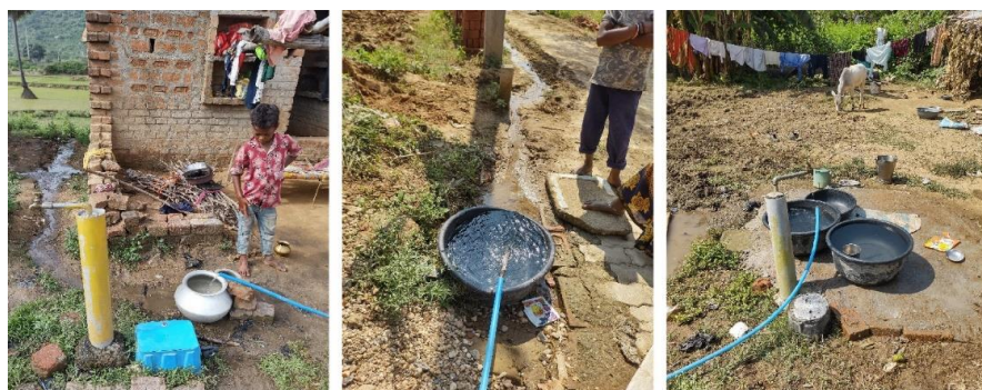
Figure 9: Broken Taps and Uprooted Pipes in Different Settlements
