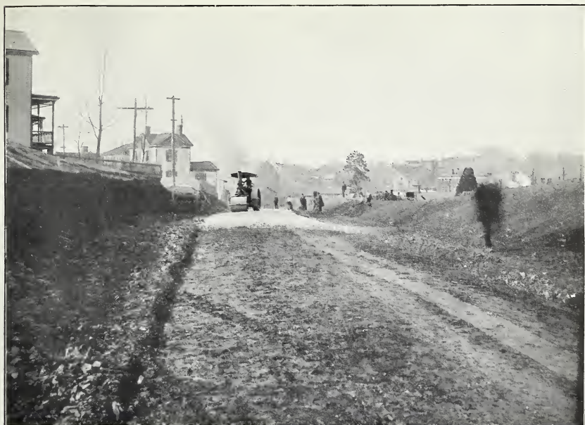
FIG. 1.—JEFFERSON MEMORIAL ROAD—PREPARED SUBGRADE, AND FIRST COURSE OF STONE.
