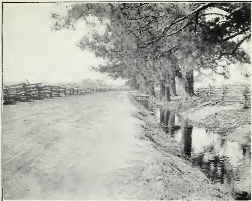
FIG. 1.—IMPROVED EARTH ROAD IN HYDE COUNTY, N. C.
