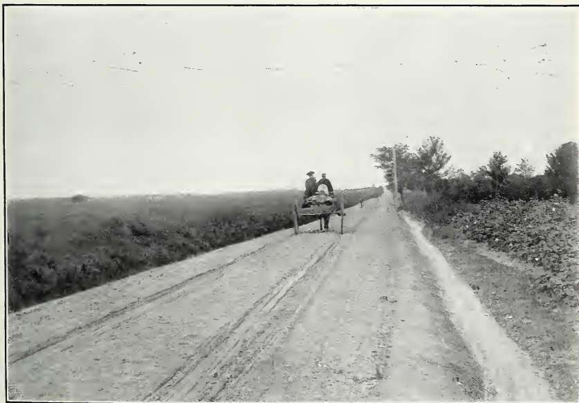
FIG. 2.—SAND-AND-CLAY ROAD NEAR NEWBERN, CRAVEN COUNTY, N. C., CONSTRUCTED AS AN OBJECT LESSON UNDER SUPERVISION OF AN EXPERT OF THE DEPARTMENT OF AGRICULTURE.
