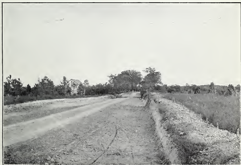
FIG. 2.—MACADAM ROAD 2 MILES SOUTH OF GREENSBORO, GUILFORD COUNTY, N. C.
