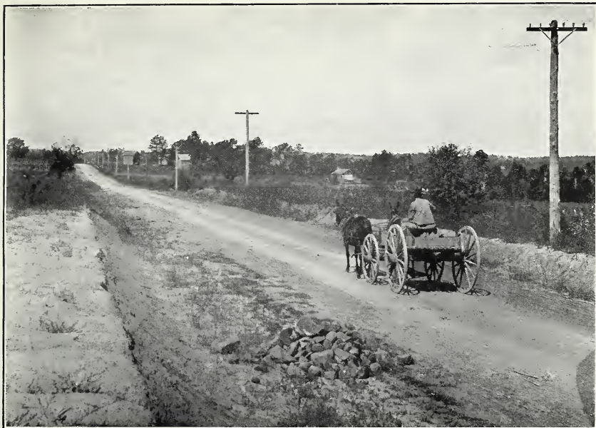
FIG. 1.—MACADAM ROAD 4 MILES WEST OF DURHAM, DURHAM COUNTY, N. C.
