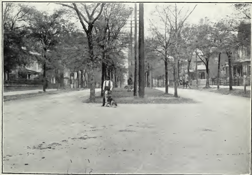
FIG. 2.—IMPROVED ROAD BUILT OF PARTIALLY DECAYED SHELL LIMESTONE, WILMINGTON, N. C.
