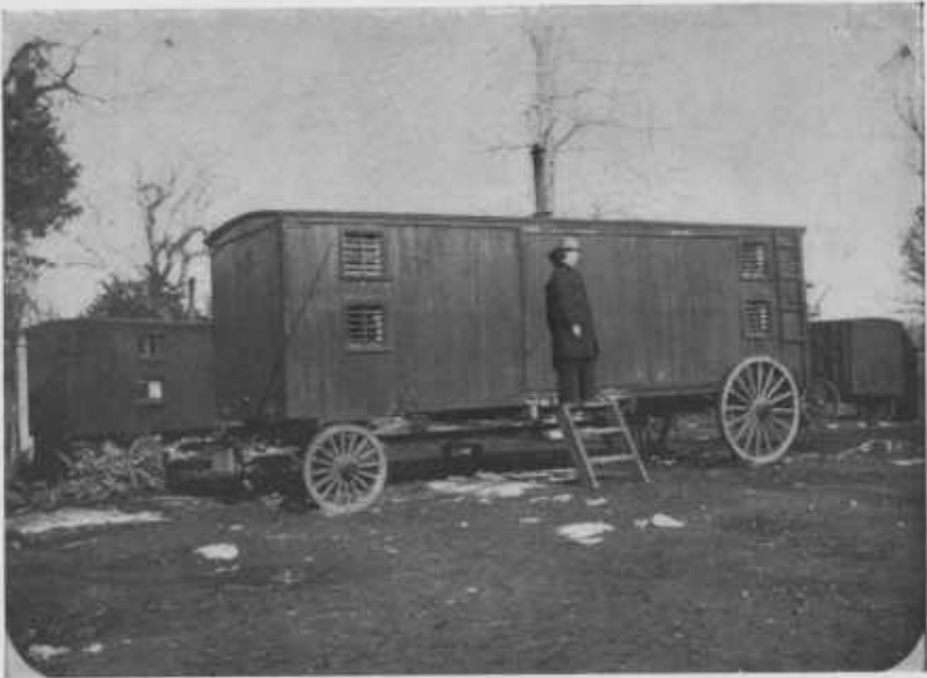
FIG. 1.—PORTABLE CONVICT QUARTERS ON WHEELS, USED FOR THE CONVICT FORCE WORKING ON THE PUBLIC ROADS IN DAVIDSON COUNTY (ABOUT NASHVILLE), TENN. [This arrangement is applicable when a small number of convicts are employed.]
