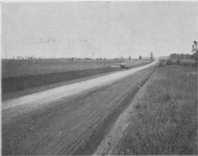
FIG. 2.—DOUBLE TRACK MACADAM AND EARTH ROAD, BUILT BY CONVICT LABOR IN MECKLENBURG COUNTY, N. C.
