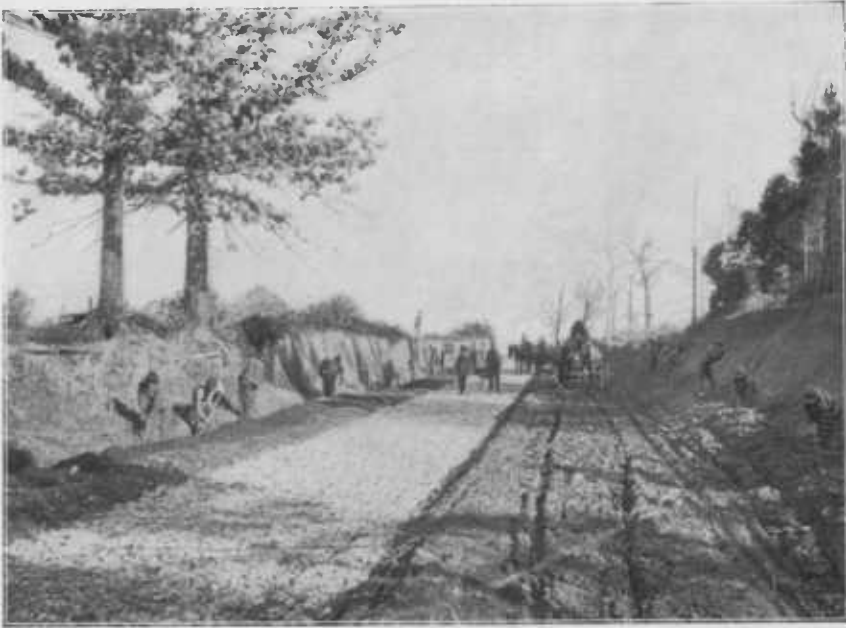
FIG. 1.—CONVICTS BUILDING A MACADAM ROAD IN MECKLENBURG COUNTY, N. C.
