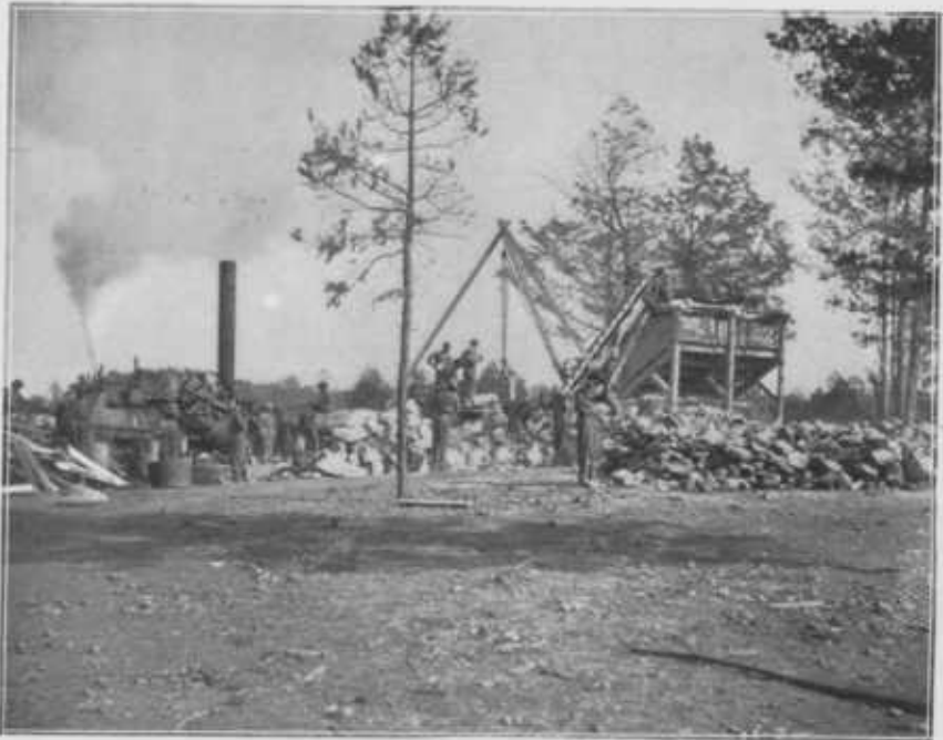
FIG. 2.—CONVICTS OPERATING THE ENGINE AND STONE CRUSHER, USED IN ROAD BUILDING IN MECKLENBURG COUNTY, N. C.
