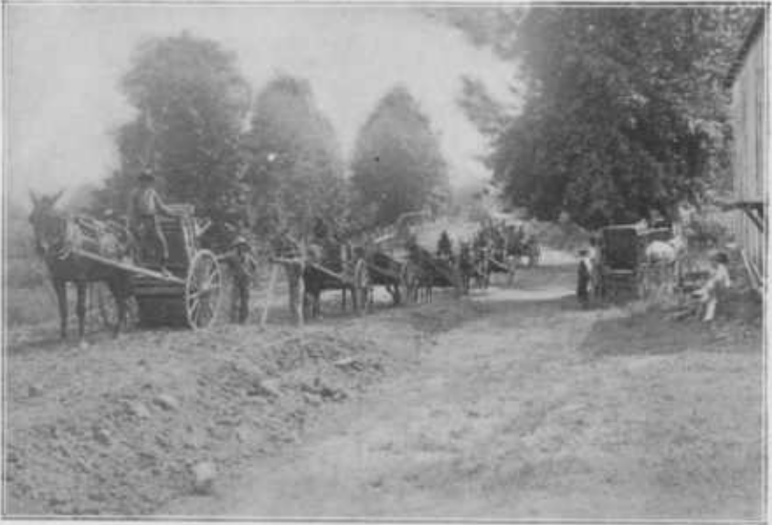
FIG. 1.—CONVICTS GRADING A PUBLIC ROAD IN SHELBY COUNTY, TENN., ABOUT 15 MILES NORTHEAST OF MEMPHIS.
