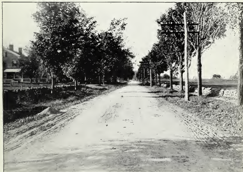
FIG. 2.—RESULTS OF REPAIRS AT SAME PLACE AS SHOWN IN FIG. 1, OCTOBER 25, 1901.
