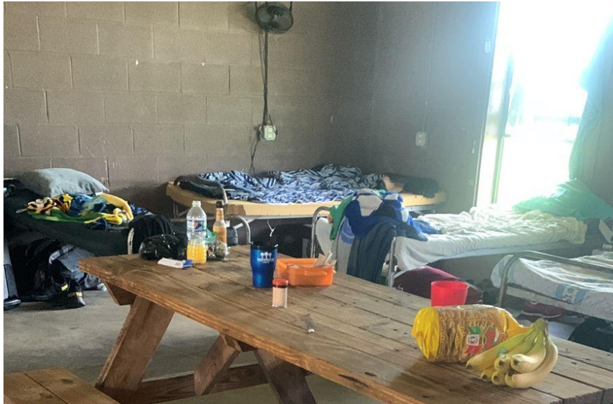
Figure 15. Farmworker Housing Conditions
