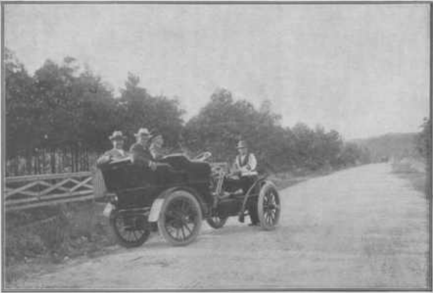
FIG. 1.—THE JOPLIN, MO. SPECIAL ROAD DISTRICT COMMITTEE INSPECTING THE FINE ROADS CONSTRUCTED OF MINING SLAG UNDER THEIR SUPERVISION. [There are about 100 miles of these roads, built at a cost of about $150,000.]
