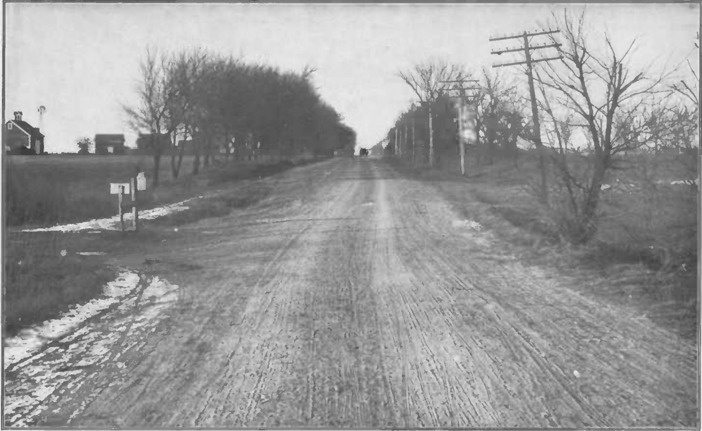
OSSEO GRAVEL ROAD, 3 YEARS OLD, 4 MILES NORTH OF MINNEAPOLIS.
