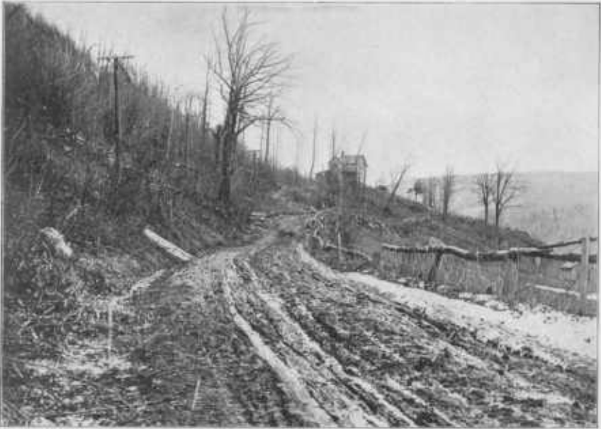
FIG. 1.—TYPE OF ROAD IN MASSACHUSETTS BEFORE IMPROVEMENT.
