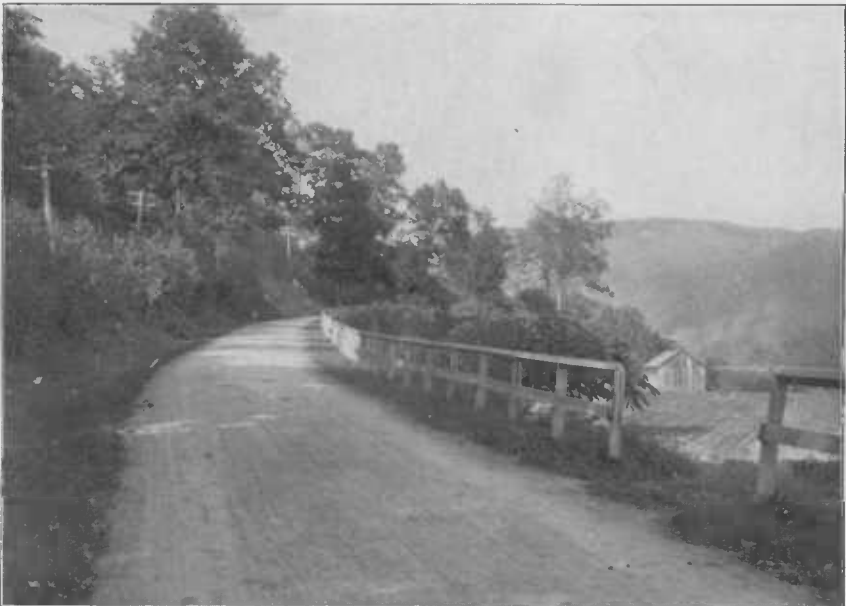
FIG. 2.—TYPE OF ROAD IN MASSACHUSETTS AFTER IMPROVEMENT.
