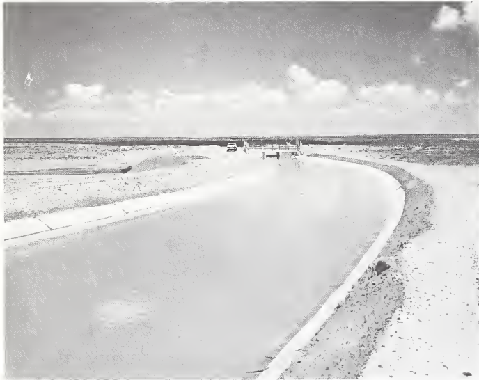
Canal at the Navajo Indian Irrigation Project, New Mexico, as the first water is being released down the Gravity Main Canal, 1977 (Photo by H. Wittman; courtesy, Bureau of Reclamation, U.S. Department of the Interior).
