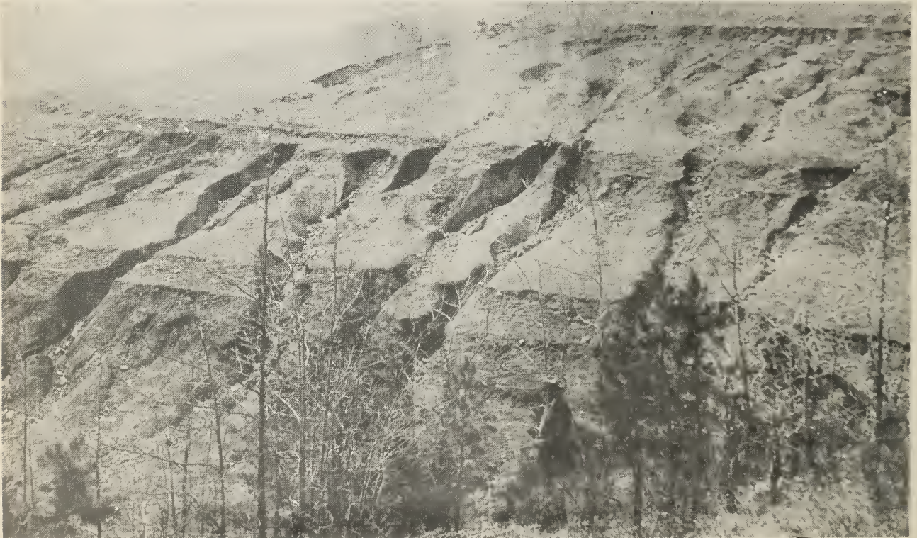
Fig. 4. When all trees were cut off this slope, erosion soon ruined the land. Silt and runoff from this hill are damaging land and property below. Some districts may wish to regulate the cutting of trees from such steep slopes to prevent future damage like this.
