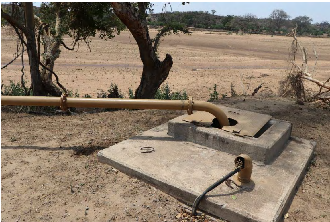
FIGURE 124: BOREHOLE IN MAPUNGUBWE CLOSE TO LIMPOPO RIVER, PUMPING WATER TO A NEARBY MINE
