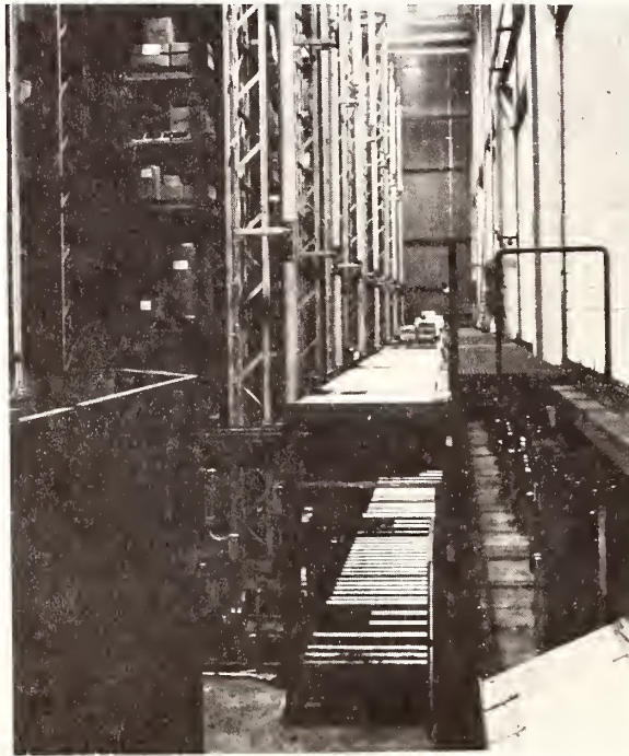
Figure 20.—A pallet load on a line roller conveyor.
