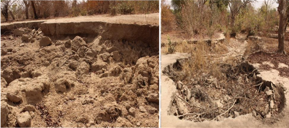
Photo 2: Gully area above the reservoir
