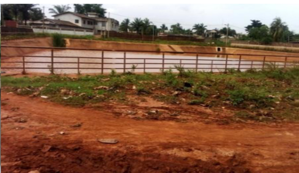
Collector leading into the retention basin in Tokpota (Porto-Novo)
