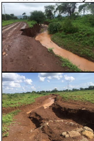
Plate 3: Erosion by surface water runoff
