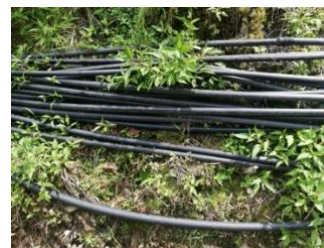
c. several HDPE hoses conveying water
