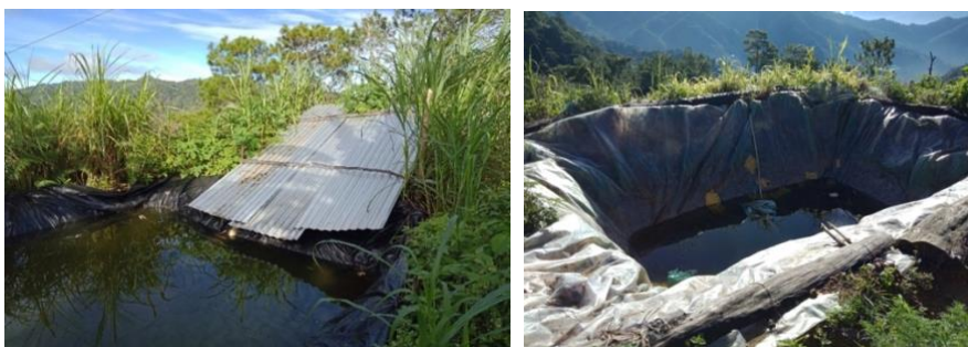
Figure 2. A rainwater or springwater harvesting embankment (4' x 8' x 5') or coilo
