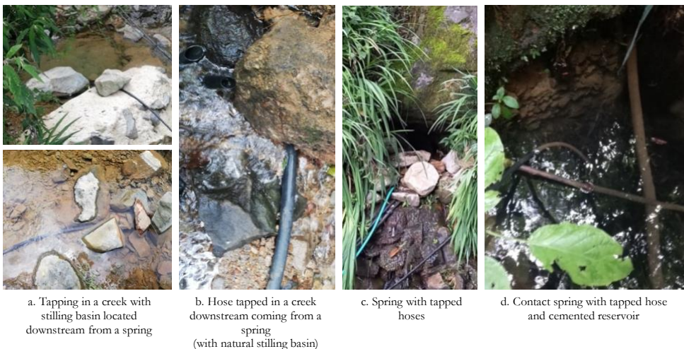
Figure 1. Tapping of hose in springs or creeks, which are the most common water source
