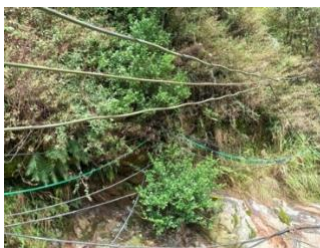
a. wires are used to support HDPE hoses
