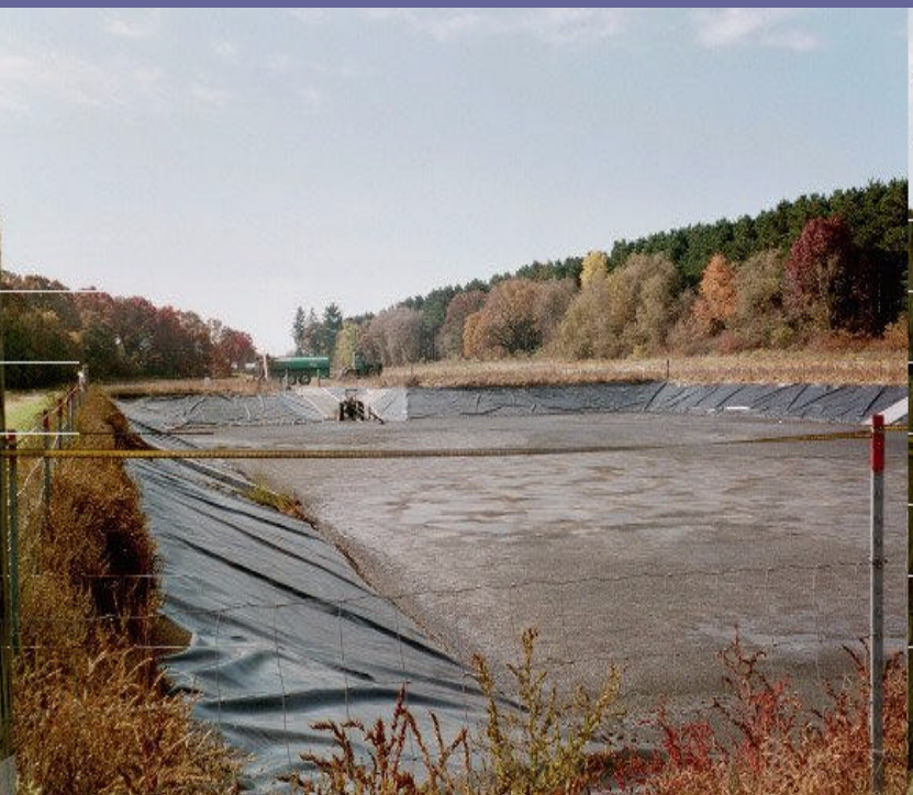
3.5 million gallon lagoon
