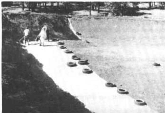
Figure 31.—Installation of asphalt-fabric, polyethylene lining in excavated reservoir.
