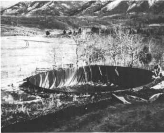
Figure 27.—Plastic-lined steel rim tank.
