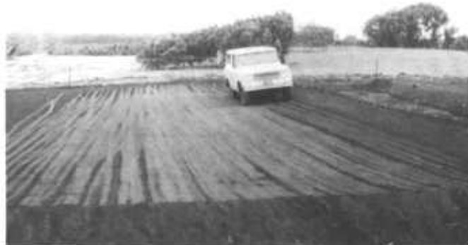
Figure 11.—Compacting a catchment apron with a rubber-tired vehicle.
