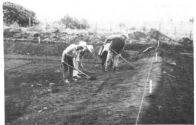
Figure 7.—Hand raking and smoothing of catchment area.
