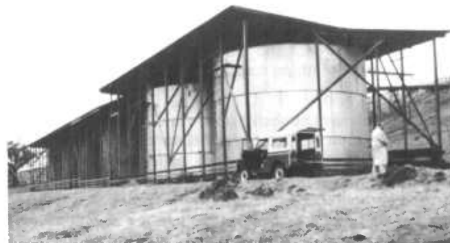
Figure 32.—Inverted roof cover over steel rim storage tanks.
