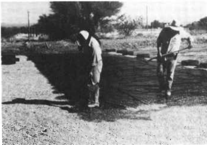
Figure 16.—Gravel placement on gravel-covered membrane catchment treatment.
