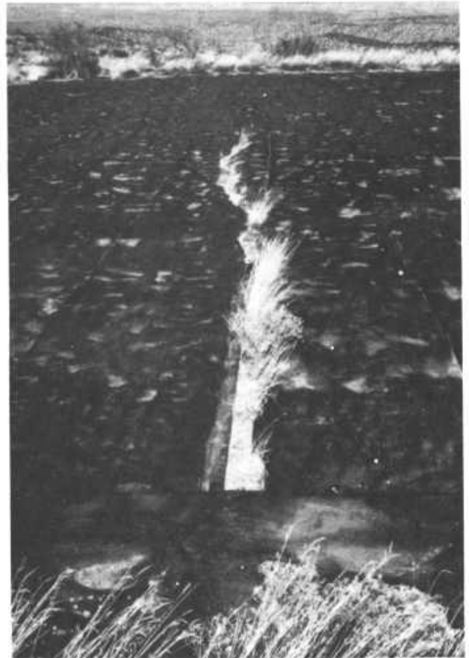
Figure 42.—Asphalt-planking catchment treatment in need of preventive maintenance.
