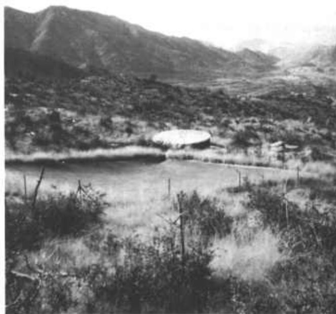
Figure 18.—Butyl rubber catchment furnishing livestock drinking water near Phoenix.
