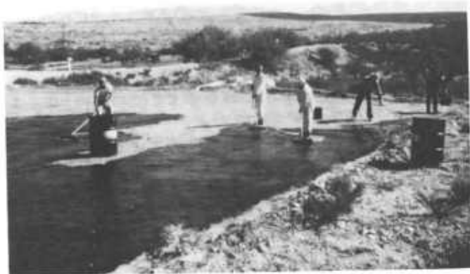
Figure 15.—Brush application of asphalt emulsion seal coat on an asphalt-fiberglass catchment.
