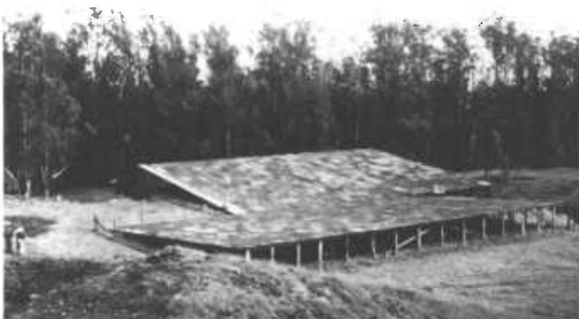
Figure 20.—Inverted V-sheet metal catchment in Hawaii.
