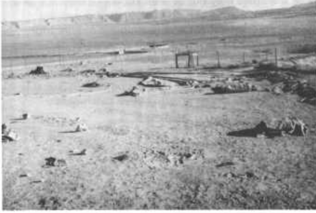
Figure 19.—Butyl rubber catchment destroyed by wind.
