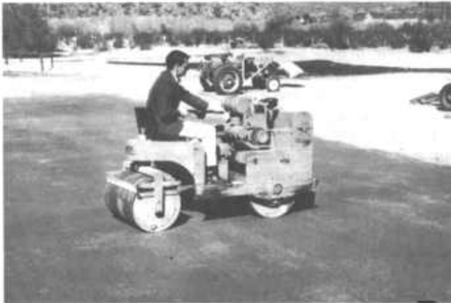
Figure 10.—Compacting a catchment apron with a self-propelled vibrating drum roller.
