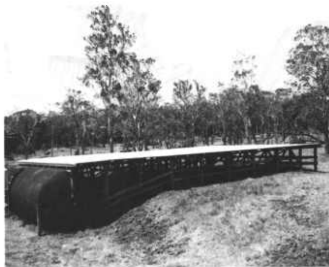
Figure 3.—Sheet metal catchment on wooden framework.
