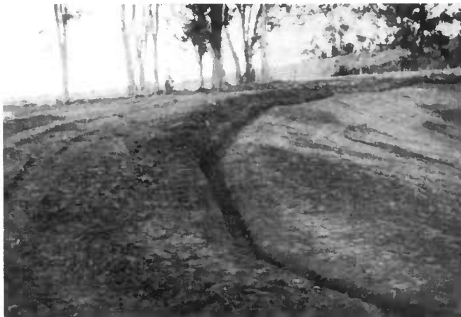
Figure 30.—Burial trench for reservoir membrane lining.
