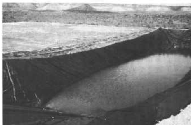
Figure 33.—Butyl-lined storage directly connected to catchment apron.
