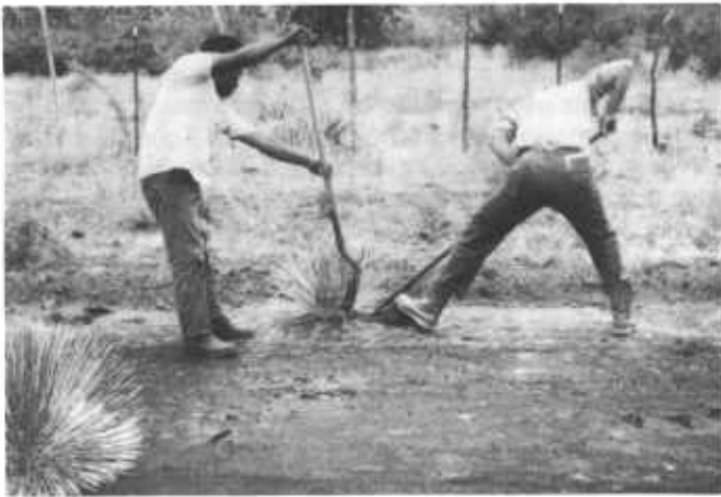
Figure 41.—Removal of plants growing through asphaltic catchment treatment.
