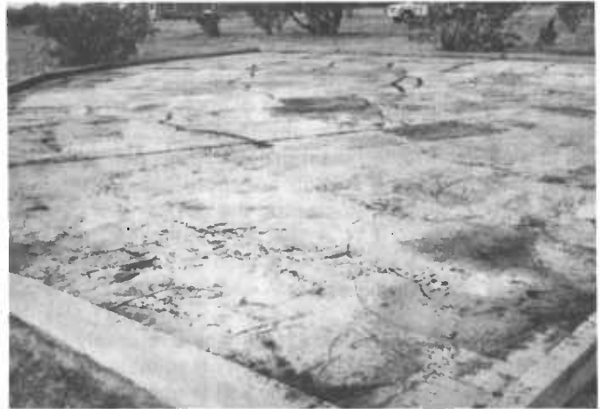
Figure 21.—Concrete catchment for wildlife water near Phoenix.
