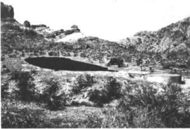
Figure 4.—Irregular shaped asphalt-fiberglass catchment matched to the natural surface topography.
