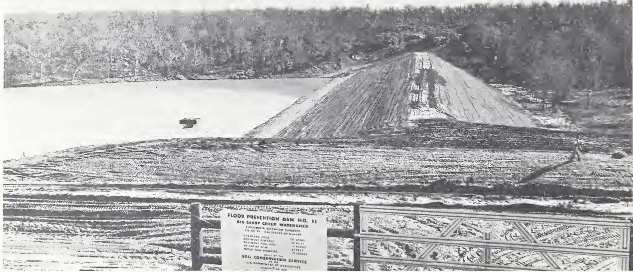
Figure 62.—Earthen dams on upstream tributaries hold back runoff water until it can be released gradually without flooding valley bottom land. In this picture, the square object in the water is the top of the drawdown tube that carries water under the dam.
