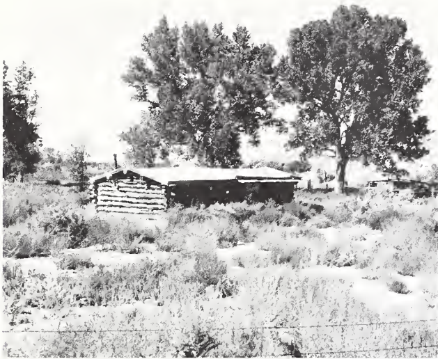
Those who found no gold began to settle the land. The sod-covered log house was the standard homesteader's residence.
