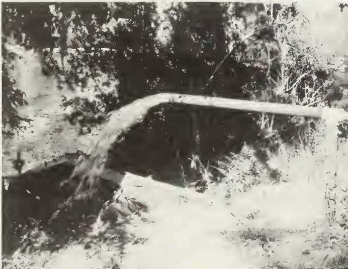
Free Flowing Well in Dougherty Plain District Discharging Water from the Principal Artesian Aquifer
