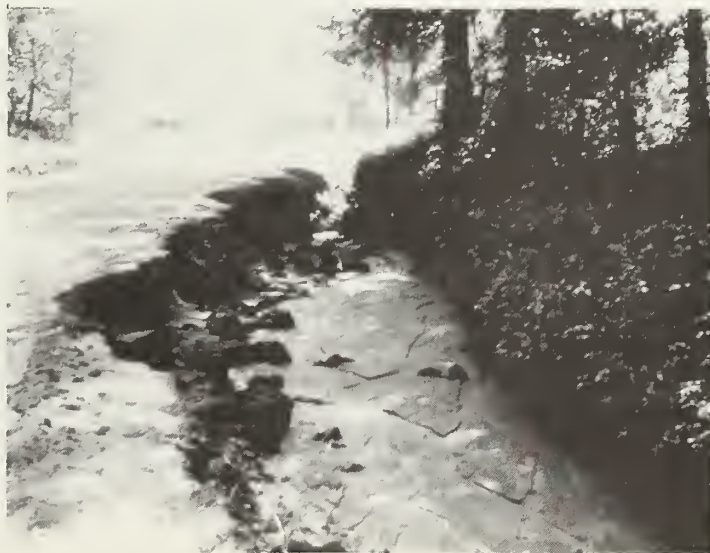
Erosion of Unstable Soils in Roadway from Concentrated Water Flow
