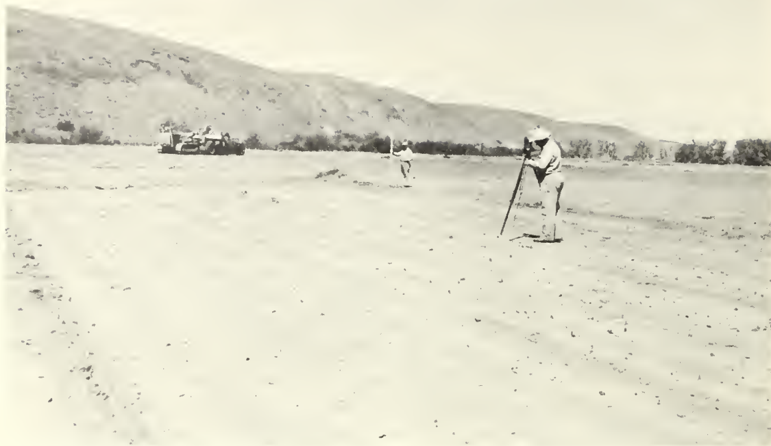
Figure 32.--Land is leveled for more efficient application of irrigation water, subbasin 3. SCS photo. 7-736-2
