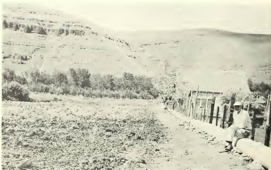
Figure 33.--A concrete pipe has been installed to replace an old wooden flume, subbasin 1. SCS photo. 7-1116-11
