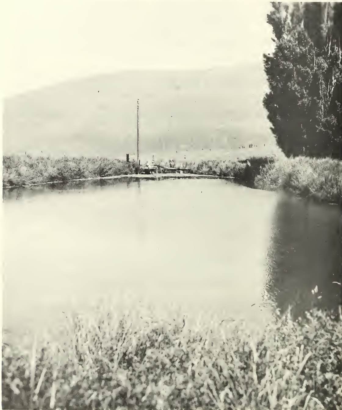
Figure 41.--A typical small reservoir constructed for multiple use in subbasin 3. SCS photo.
