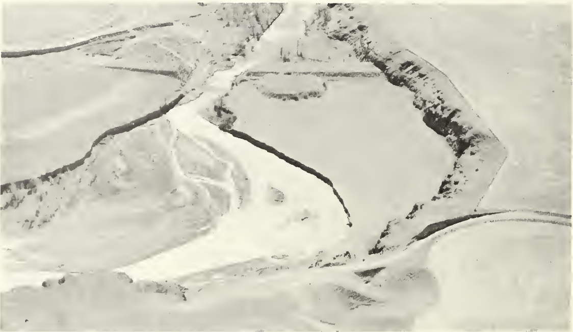
Figure 31.--Furnish Reservoir was abandoned due to sediment after 22 years. Alluvial fill in the old reservoir is now being cropped and in turn eroded away by the Umatilla River, subbasin 2. SCS photo.
