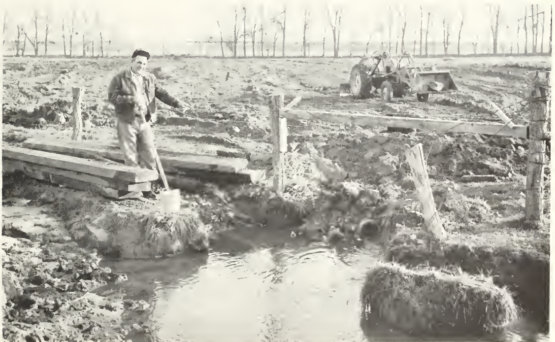
Figure 35.--Tile drainage system is newly installed to drain land in subbasin 2. SCS photo. 7-1077-7
