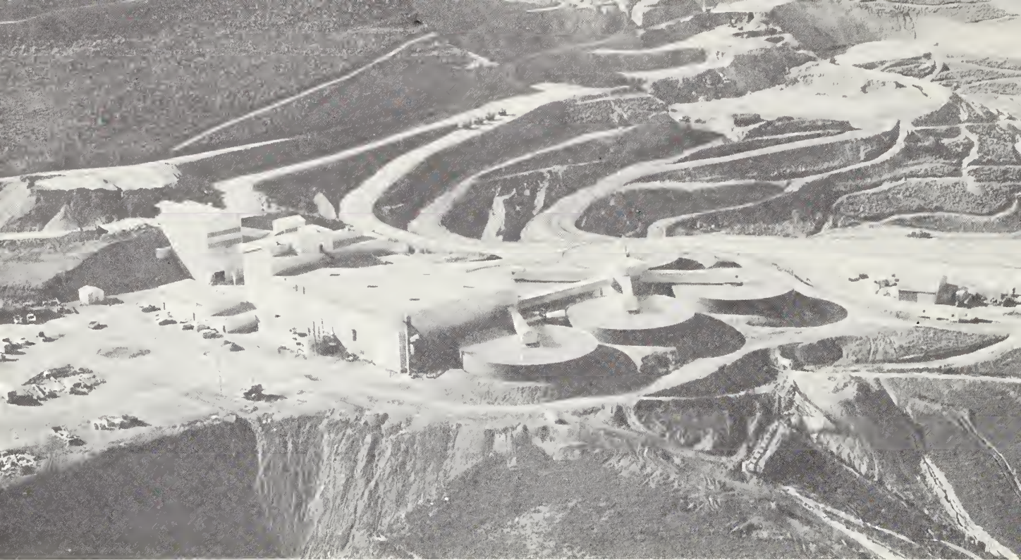
Photograph 7. - Aerial view, ore-reduction mill of the Carlin Gold Mining Company, a subsidiary of Newmont Exploration, Limited. The mill is located on the Maggie Creek-Boulder Creek divide, about 10 miles north of Carlin, on the divide between Maggie Creek and Battle Mountain Sub-Basins.
