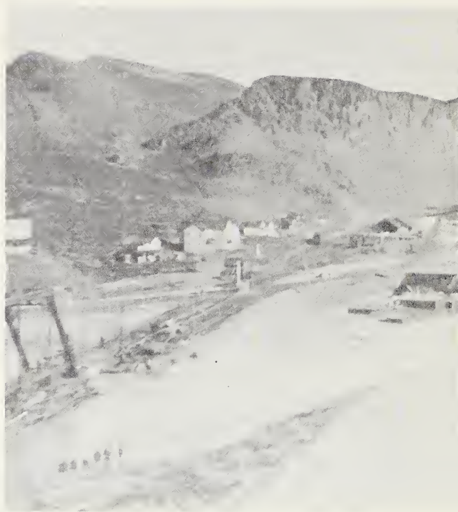
Photograph 59. - At Palisade the river swamped the Eureka & Palisade railroad yards, the south section of the town, and washed out the recently completed Southern Pacific railroad bridge, among other damages, 1910.
