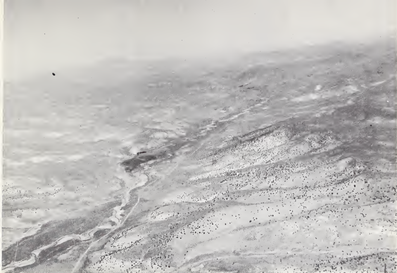
Photograph 78. - The constriction of the Susie Creek bottomland seen in the middle distance of this aerial view marks the site of a proposed Public Law 566 structure.
