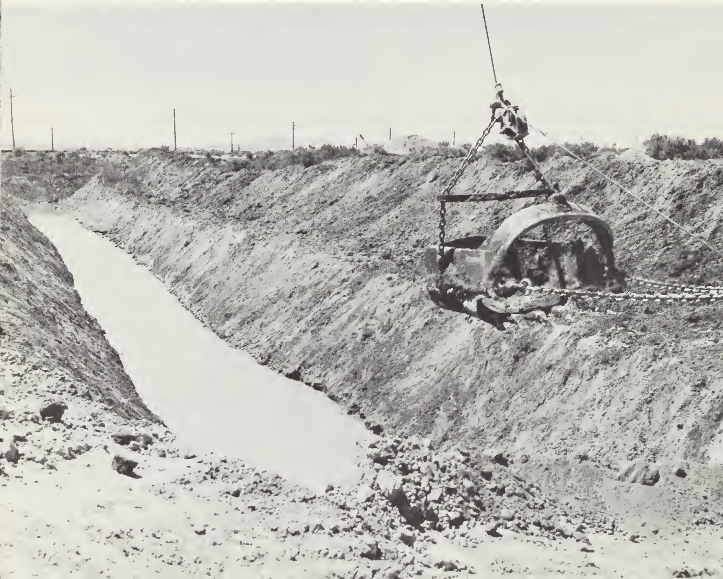
Photograph 57. - Digging a deep drain by dragline, lower Lovelock Valley; Lovelock Sub-Basin.
