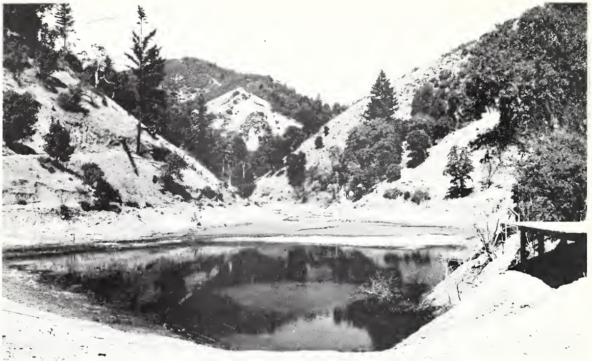
Babe Woods Irrigation Dam, Dry Creek Watershed, Mendocino County. The delta formed by sediment deposits substantially limits the water storage area.
