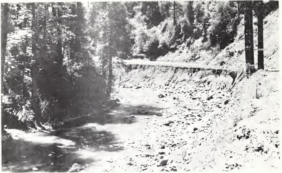
Salmon Creek near Myers Flat, California. Road encroaching on stream causing erosion.
