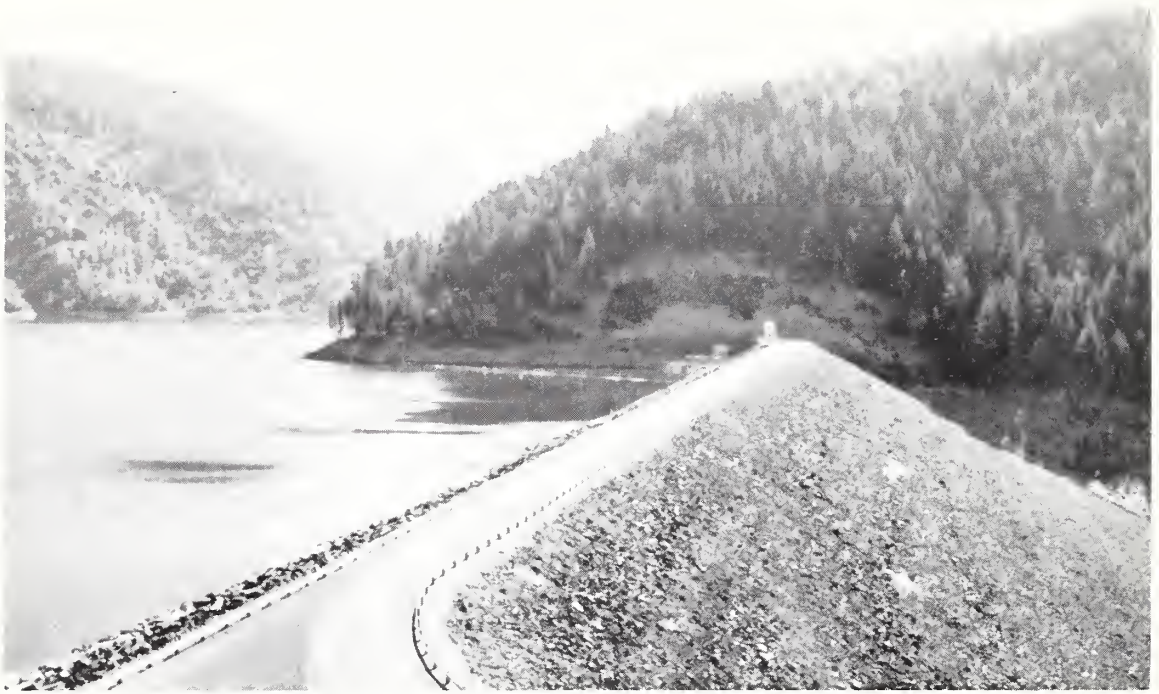
Trinity Dam, 30 million yard earth fill dam, 1/2 mile long and 1/2 mile wide at the base.
